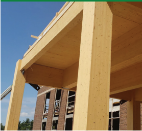
Glulam Beams & Columns
