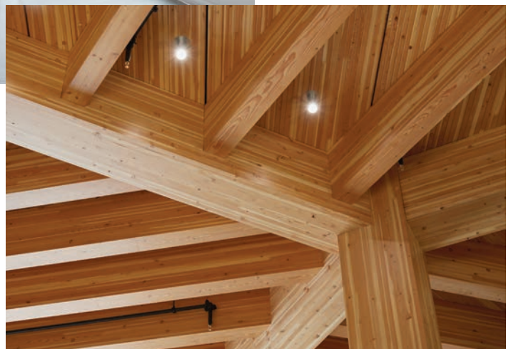
NLT ceiling with glulam beams and columns at Wellesley College Science Complex in Wellesley, MA Skidmore Owings & Merrill / Le Messurier
