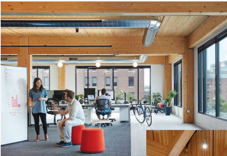
NLT ceiling with glulam beams and columns at T3 Minneapolis in Minneapolis, MN MGA – Michael Green Architecture / DLR Group / Magnusson Klemencic Associates / StructureCraft
