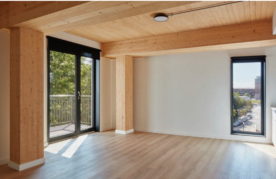
CLT ceiling with glulam beams and columns at 11 E Lenox in Boston, MA Monte French Design Studio / H&O Structural Engineering
