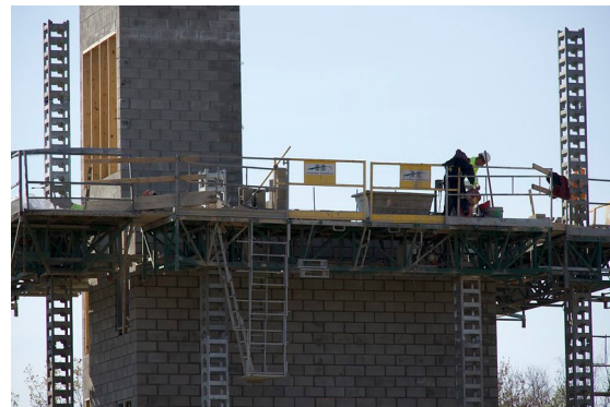
American House Meridian Elevator Construction
