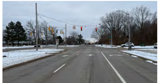
Southbound Hagadorn Road at Hannah Boulevard
